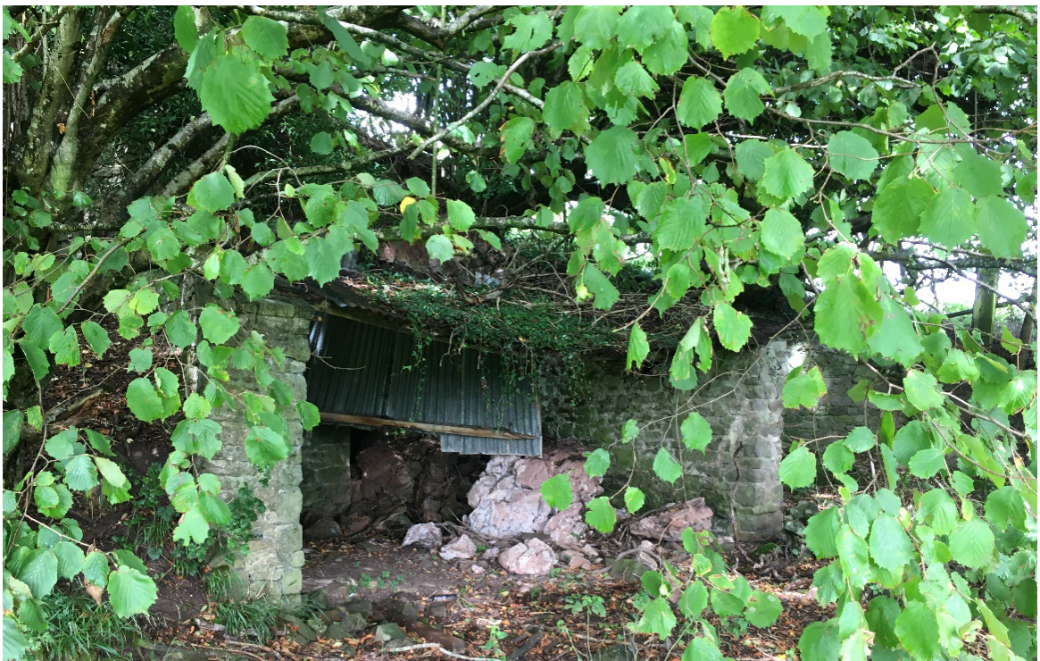
Figure 3.4: Lime Kiln, taken 24.08.20.
