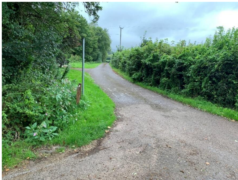
Photograph 2: The Site Access Track
